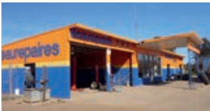
Beaurepairs Finley, NSW
